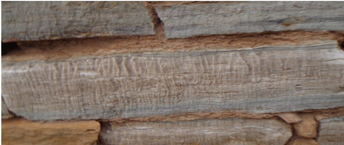
Figure7. This is one of the longest of the marble stones, which the masons significantly used to construct the Mosque. The stone slab measures about 1.3 meters long. The lime mortar firmly bounded the stones. Photograph by the researcher.
