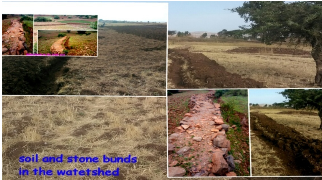
Figure 4. Soil and stone bunds constructed by the community in the study area
